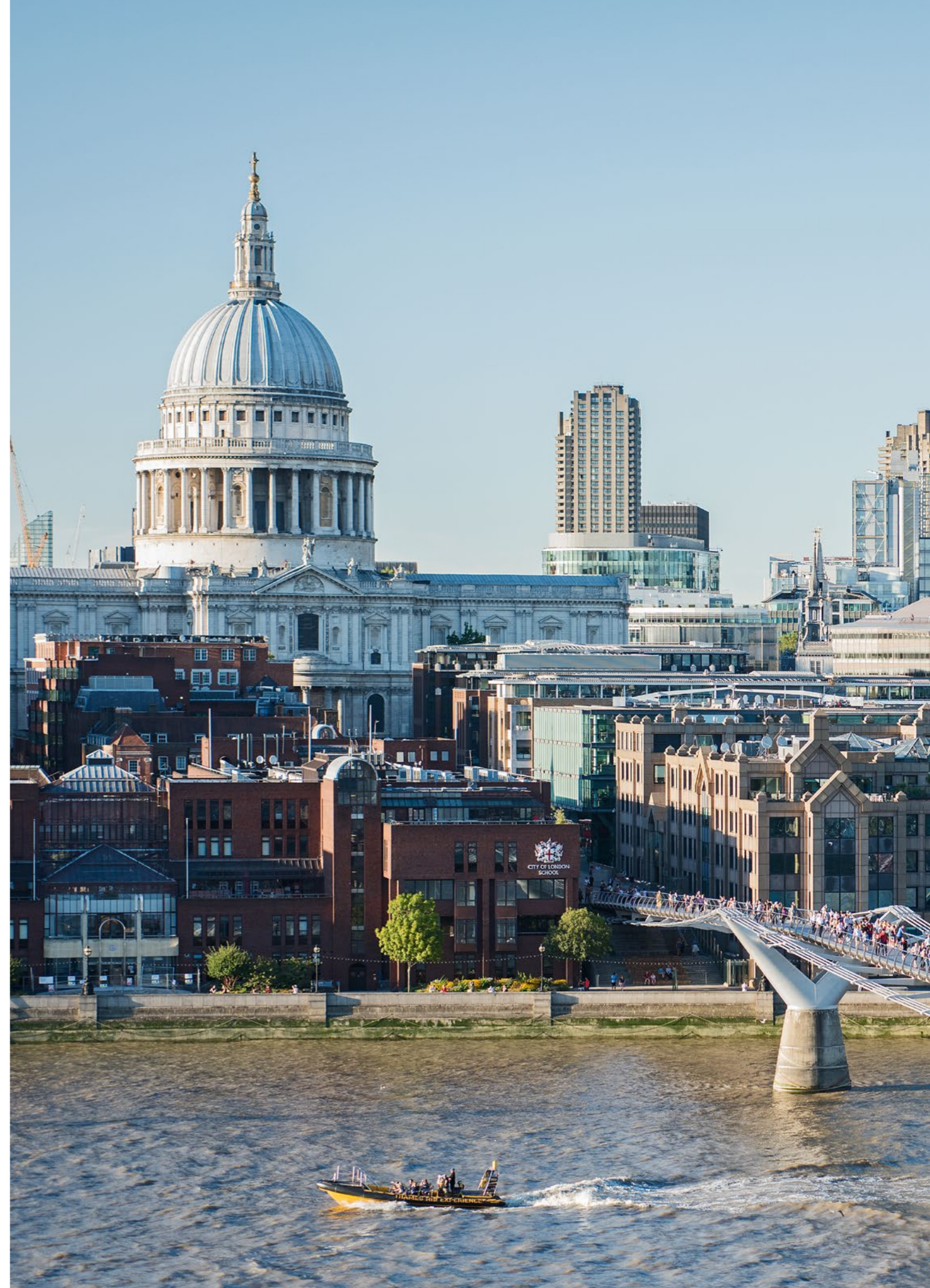
Work is ongoing to address water ingress issues at St Paul's station
